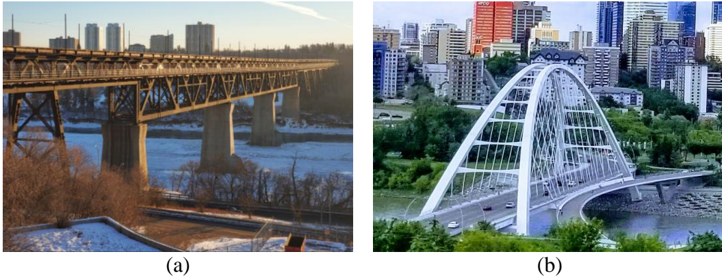
Figure 9. Pictures of (a) High Level Bridge and (b) Walterdale Bridge.
